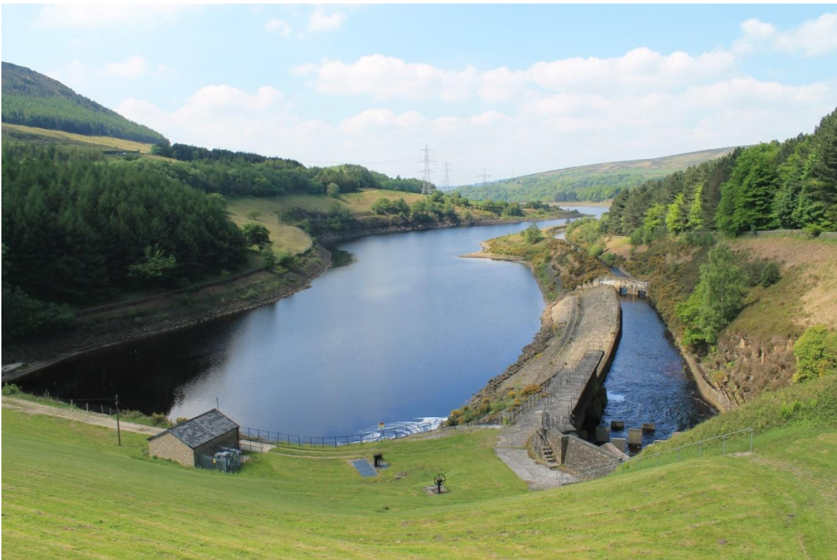
Rhodeswood Reservoir, looking west
