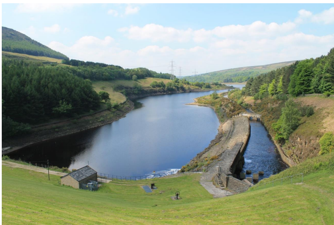
Rhodeswood Reservoir, looking West
