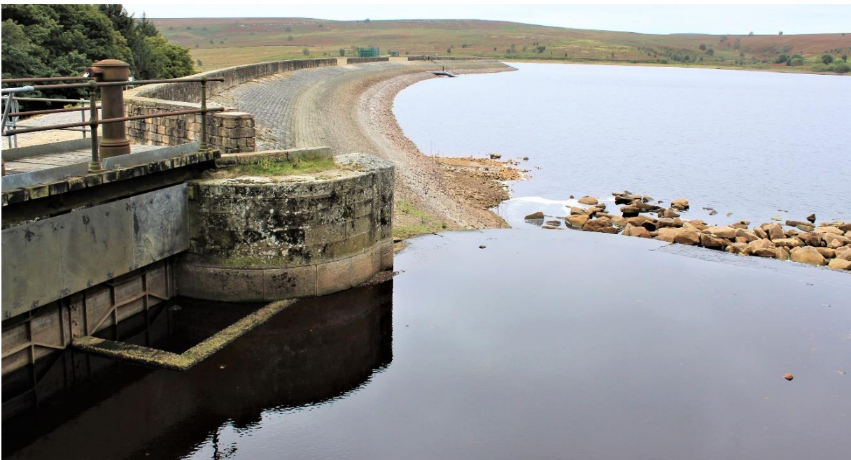
Redmires Upper Reservoir dam wall (11)
